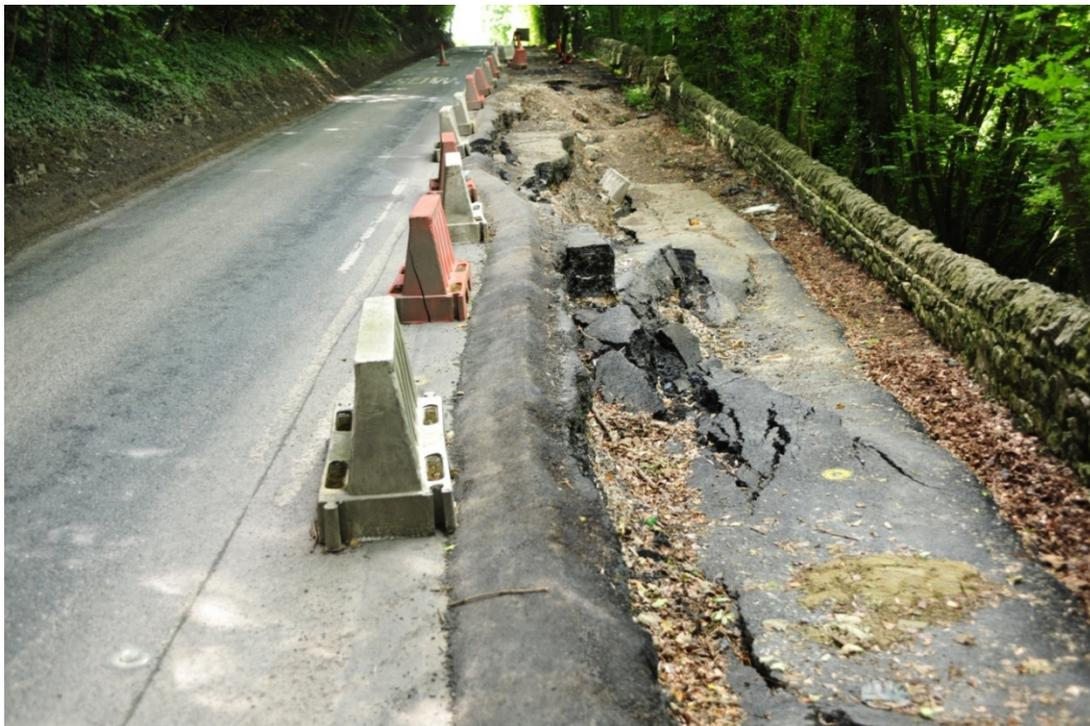
Damage to the B5056 road caused by the reactivation of part of the existing landslide
